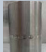
Pipe butt weld Ø 31.75 x 2 mm
