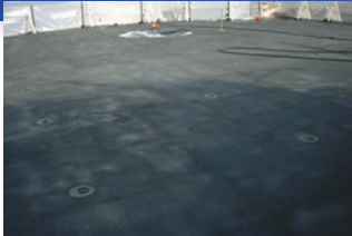
Flight deck – First full coat of Jota Armour
