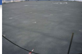
Flight deck – Second full coat of Jota Armour
